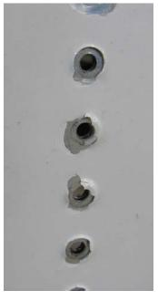
FIGURE 2: RIVET HEAD PAINT BUILDUP
