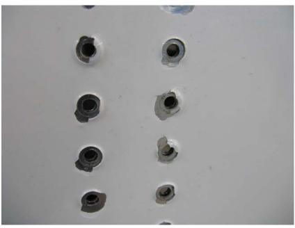
FIGURE 7: RIVET HEAD PAINT BUILDUP
